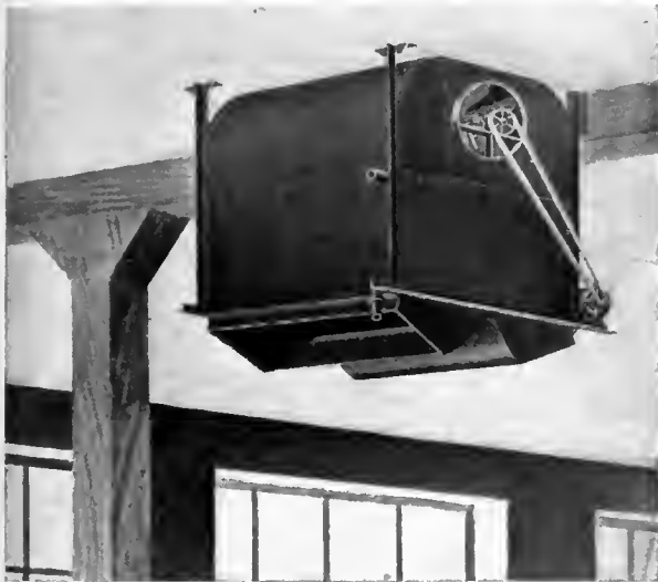
FIG. 11. TYPE OF UNIT HEATER SUSPENDED FROM CEILING
